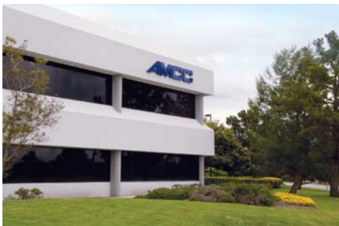
AMCC Headquarters in Sunnyvale, CA
